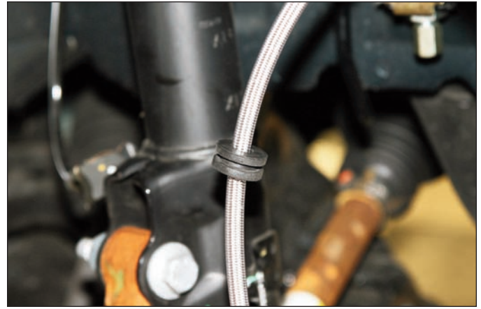
Sequence 22: Slice a grommet so that it can be slid over the Wilwood flexline that is already attached to the hard line. Install into the OE bracket and attach bracket using OE bolt in original location. Secure line as necessary to prevent contact with moving suspension, brake, or wheel components. Bleed the system referring to the additional information in the data sheet as necessary for proper bleeding instructions.
